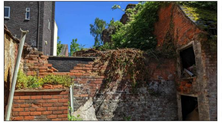
Photo D Existing outbuildings and garden wall
