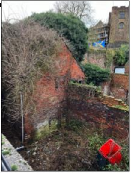
Photo B Existing outbuilding and garden wall with castle wall behind
